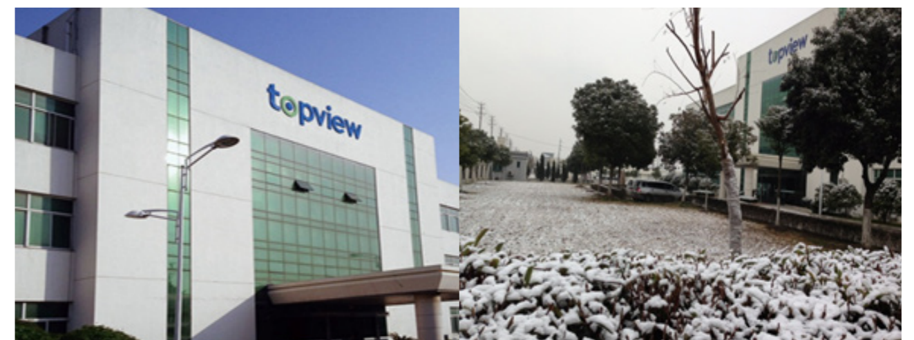
▼ 大陸昆山廠 Kunshan, China Manufacturing Plant
